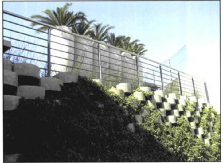
Retaining wall between a children's play area and a staff function area on the upper level
